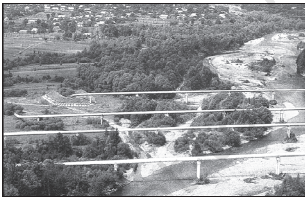
Fig. 7.17: Pipelines transporting natural gas in Ukraine
