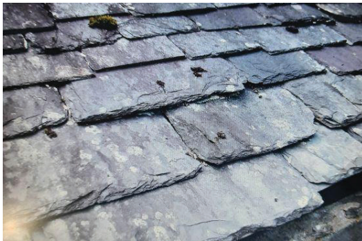
Fig. 11.6: Rocks used for roofing
