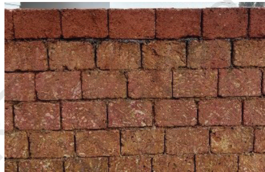
Fig. 11.7: Laterite rocks used as bricks
