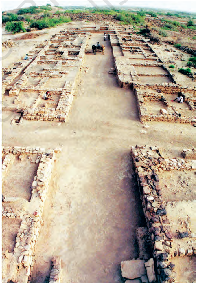
(Right) Fig. 6.5. Housing area in Dholavira, with perpendicular streets, in the middle town (Dholavira had three distinct zones, not two as in other cities). Also, in this city, the foundations of most buildings were made with stones.
