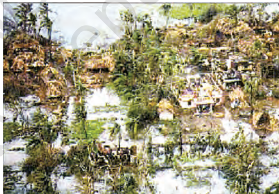
Destruction caused by a cyclone
